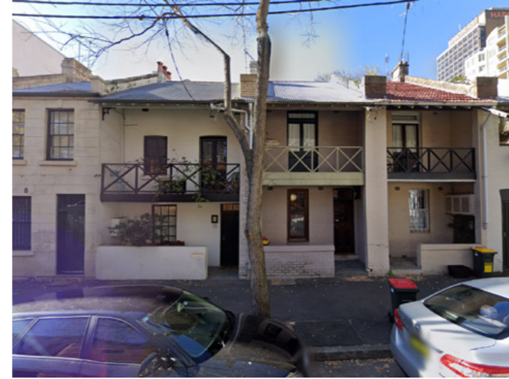
Cathedral Street Character Area, terraces on Riley Street
