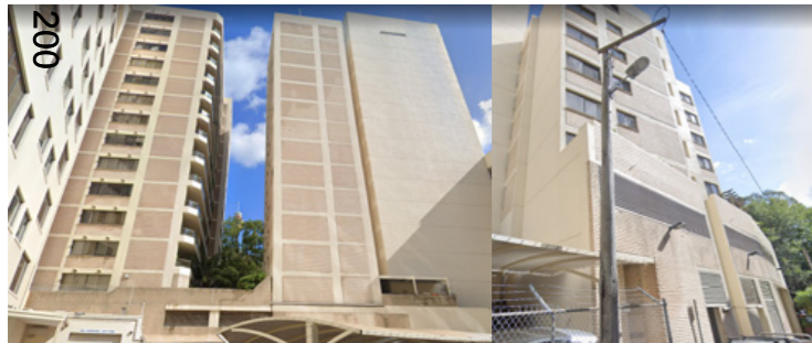
Servicing William Street
