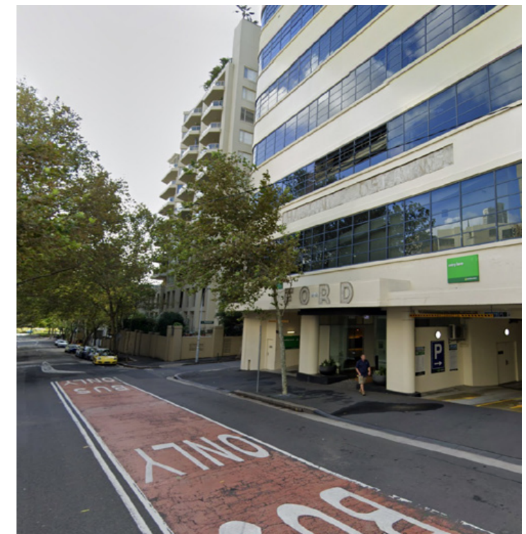
Riley Street, looking northeast towards Ford building
