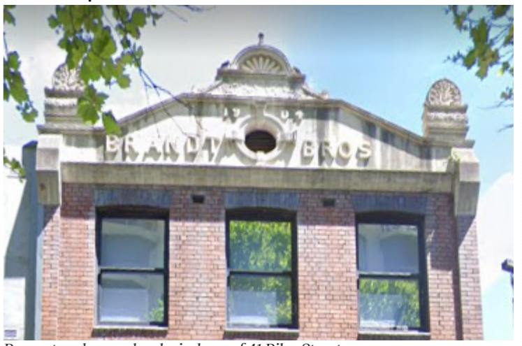
Parapet and upper level windows of 41 Riley Street
