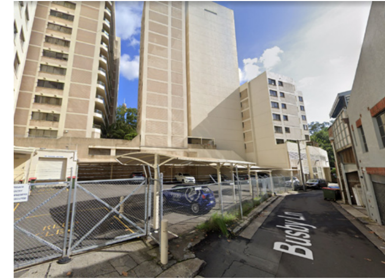
Busby Lane, looking west towards car park of residential development
