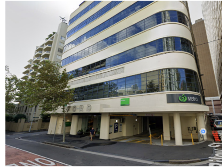
City Ford Building, Riley Street
