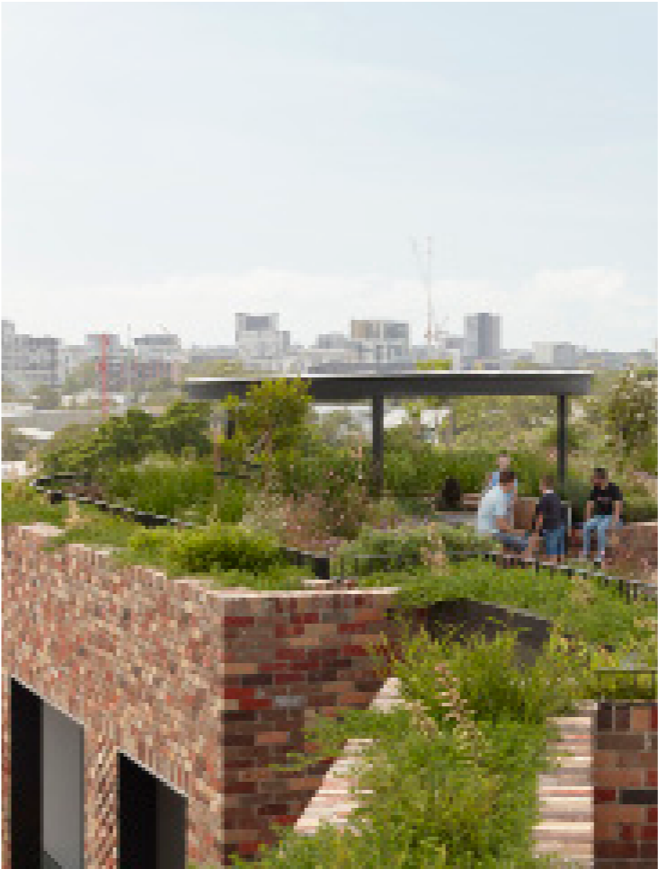
Green roof, Arkadia DKO
